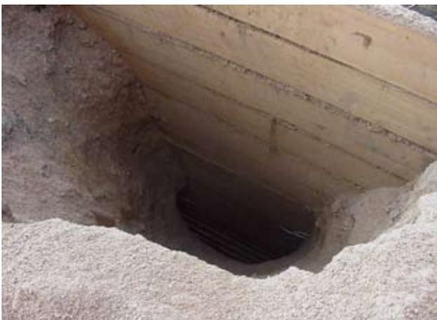
[FIG. 9] Soil Silo Formed by Caving (Courtesy of Coggins and Sons, Inc.)
