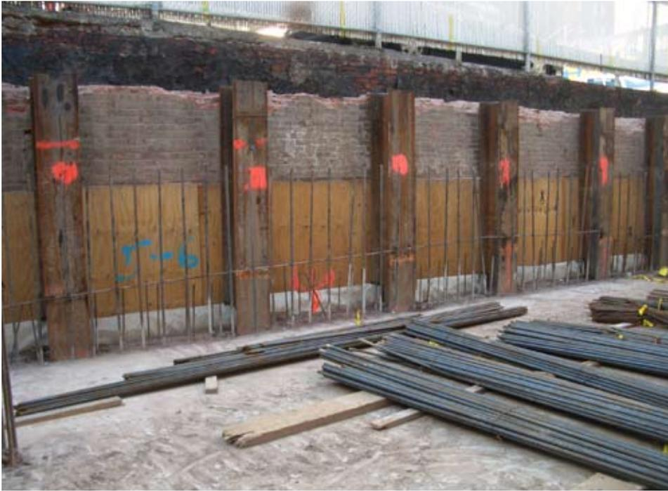
[FIG. 8] Existing Brick Wall Used as Lagging
