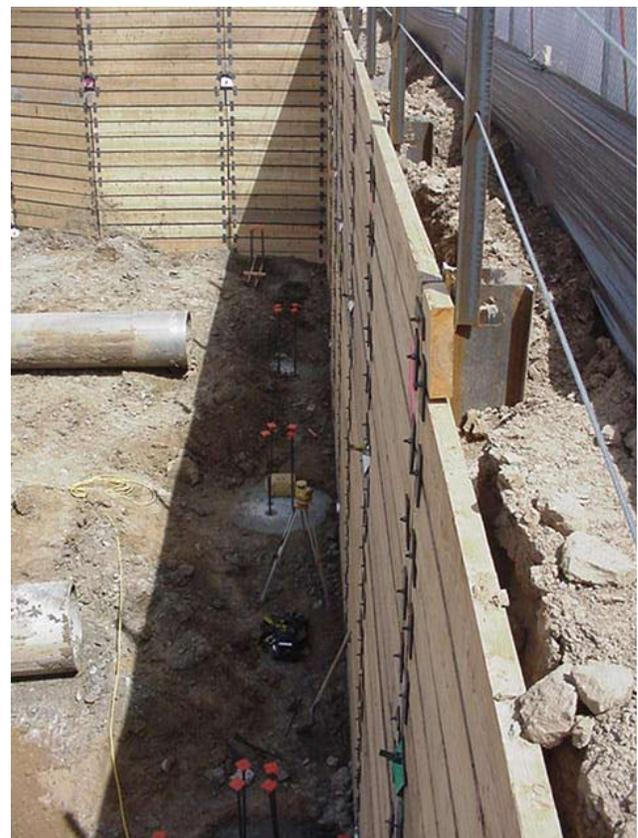
[FIG. 10] Separation Between Lagging and Cohesive Soils (Courtesy of Coggins and Sons, Inc.)
